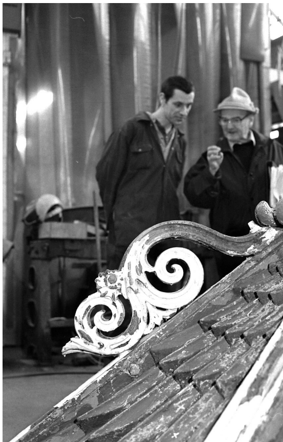
Theo Williams checking up on the repairs to the cast iron roof and columns of Beckford's Tower during a visit to Dorothea Restorations in Bristol, 1998.
